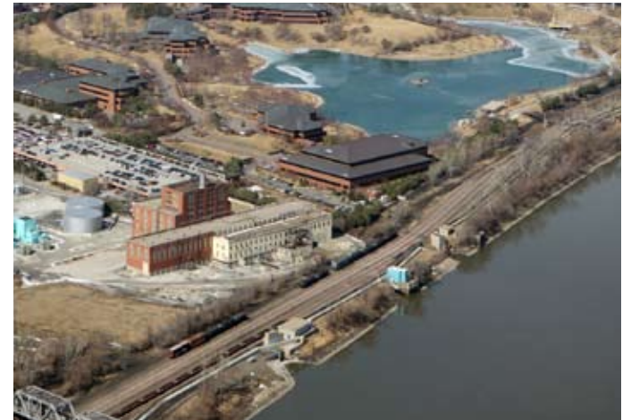
Riverfront railroad tracks do not allow direct connections to the River
