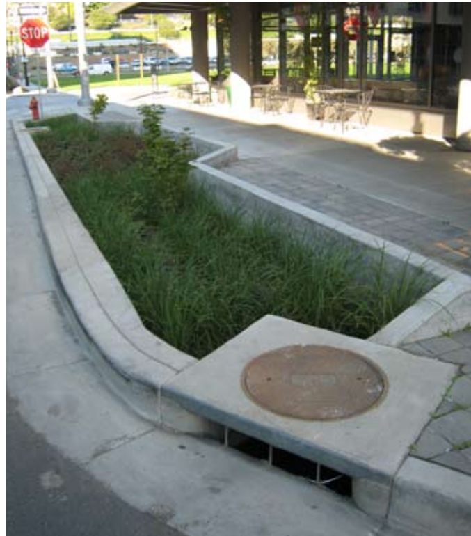
Curb-side swales can be used in dense urban environments to increase stormwater absorption and add landscaping
