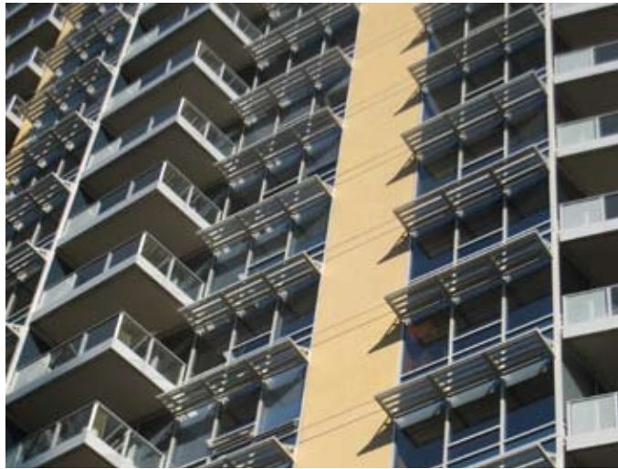
Climate sensitive features like these sunshades can be a feature of high quality design projects.
